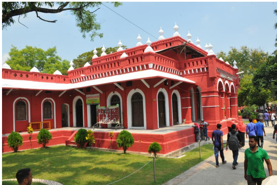
Gallery building erected by the financial aid of Haji Muhammad Mohsin (former Madrasa building)
